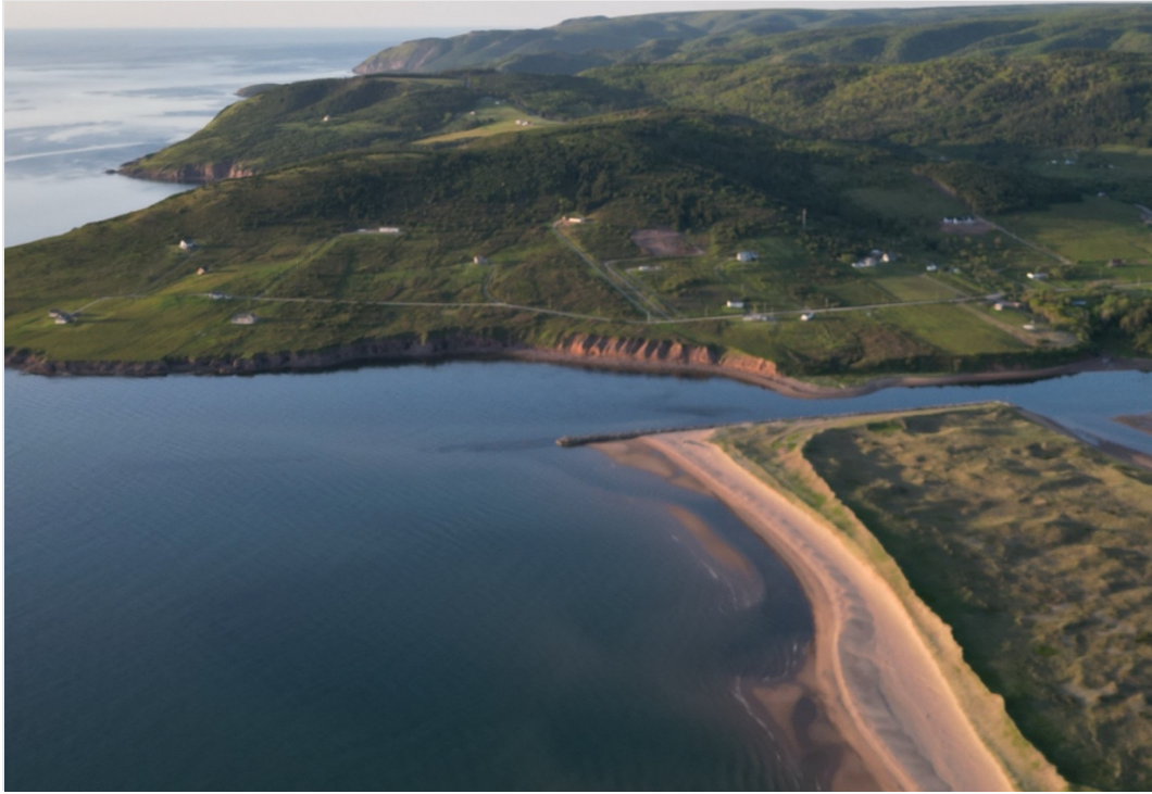
Figure 8. Aerial view of the Outer Mabou Harbour Breakwater.
